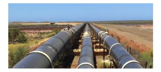
Horizontal pipeline (only friction losses), length 200 km, is pressure is 20.000 kPa
