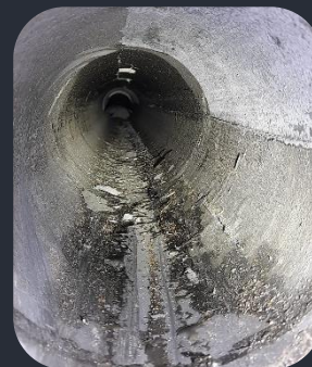
Scaling: Accumulation of scale on the internal walls of the pipeline.
